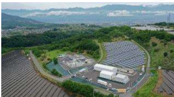
1.5MW PEM electrolysis (Yamanashi Hydrogen Company)
